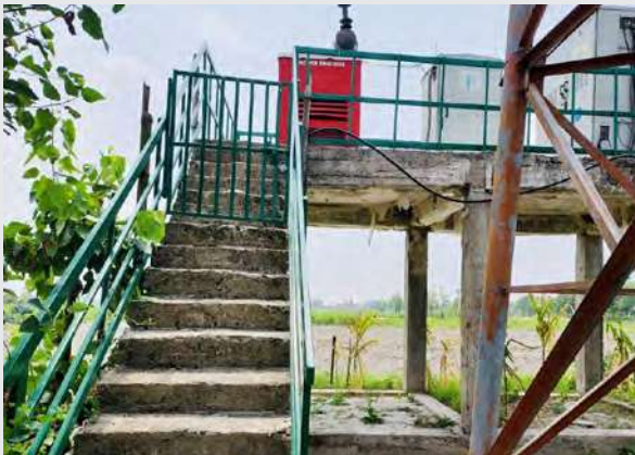
Infrastructure elevated to combat flood impact
