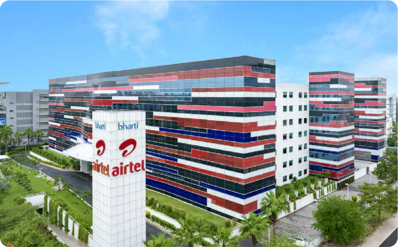
Airtel Center, Gurugram received Advanced certification under Excellence in Design for Greater Efficiency (EDGE)
