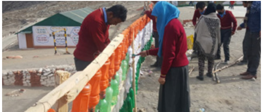
Students of Army Goodwill School Harka Bahadur built a protective boundary wall by reusing waste plastic bottles in Kargil, Ladakh. The project featured among 'Top Four' in Design for Change.
