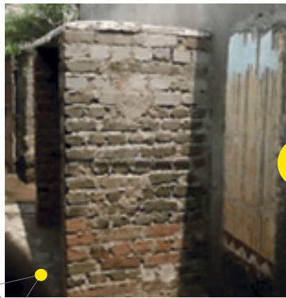
Situation before construction and installation of WASH related infrastructure
