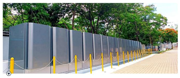
Solid oxide fuel cell based hydrogen-ready power plant at Bengaluru DC
